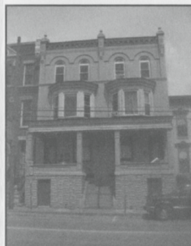
#6 Johnson Apartments 738-740 Main St
