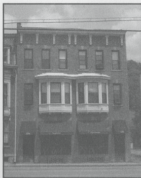
#1 Sauter Apartments 836-838 Main St
